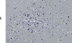
Continue rolling out approximately 6 foot wide sections and tossing chips until the entire floor is complete. Since everyone's idea of chip coverage can be different, it's important to make sure you don't run out of chips before
